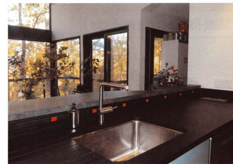
Photo: Larry Palmer Black epoxy resin countertops at the sink and Honduras mahogany trim around the windows complement the industrial theme of the space.
