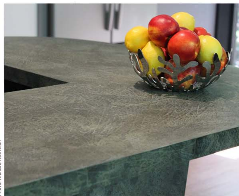
Photo: Richard Rothwell Larry Palmer acid-etched 22-gauge zinc plating to create the desired color, pattern and patina.
